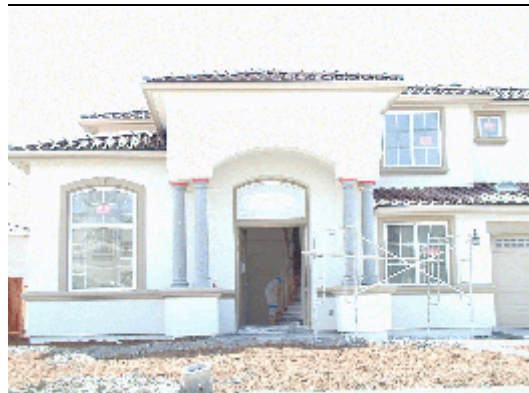
Home at Ponderosa Cove under construction
