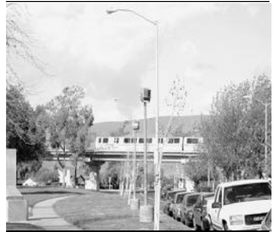
Elevated BART tracks on Decoto Road
